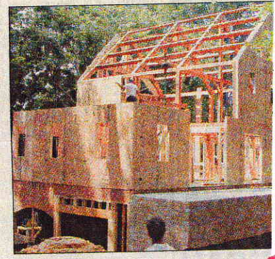
The southeast corner of Kim and Pat Kasdorf's home, above, has a roof overhang, 6 feet, 8 inches at the peak, that shades all but the lowest level of windows on the porch, thus greatly reducing solar heat gain in mid-summer. The Kasdorf's home under construction, right, reveals the timber frame structure as well as the structural insulated walls. The SIP walls and roof provide extremely high R value rating.
