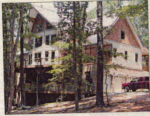
The southeast corner of Kim and Pat Kasdorf's home, above, has a roof overhang, 6 feet, 8 inches at the peak, that shades all but the lowest level of windows on the porch, thus greatly reducing solar heat gain in mid-summer. The Kasdorf's home under construction, right, reveals the timber frame structure as well as the structural insulated walls. The SIP walls and roof provide extremely high R value rating.
